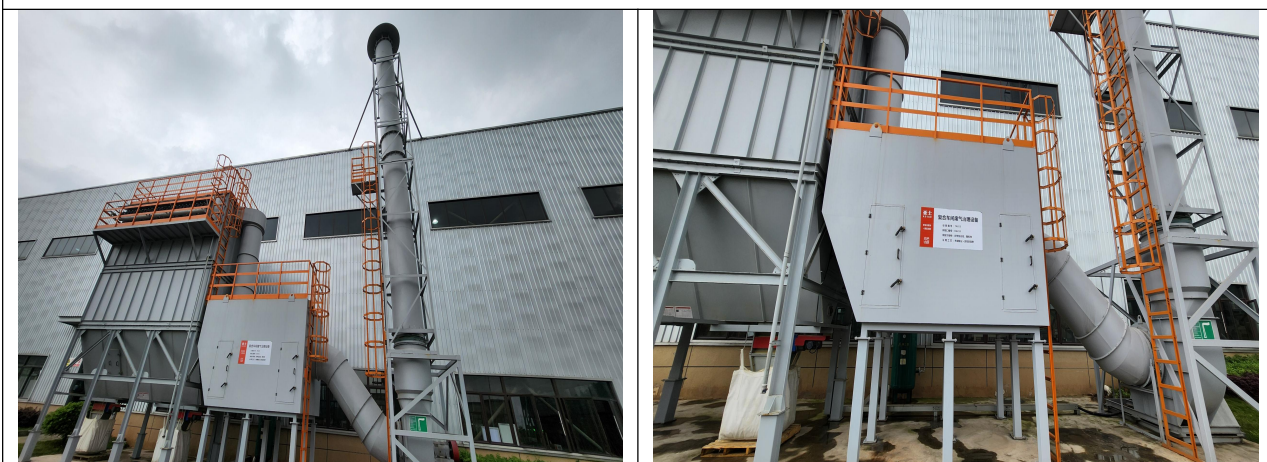
复合线上板粉尘、涂胶等有机废气
